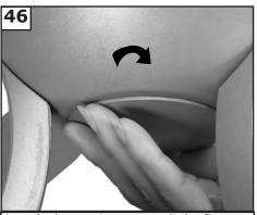
Attach decorative cap to light fixture by twisting into place.
